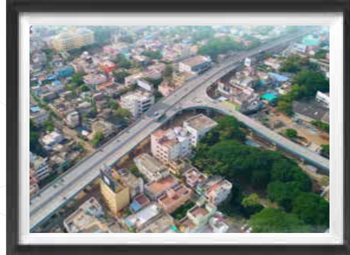
Flyover on NH45A PUDUCHERRY
