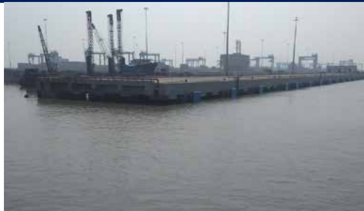
Coastal Berth at JN Port, Mumbai
