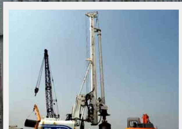
Hydraulic Piling Rig
