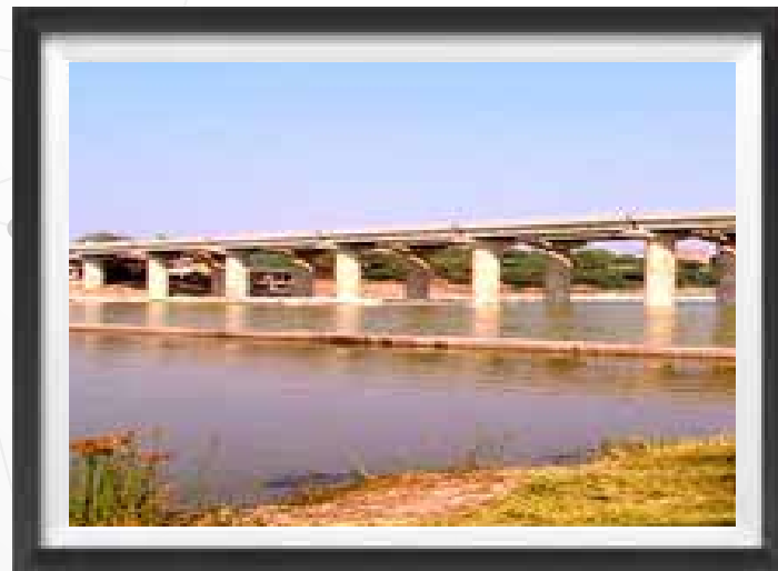
Bridge on River Godavari NANDED
