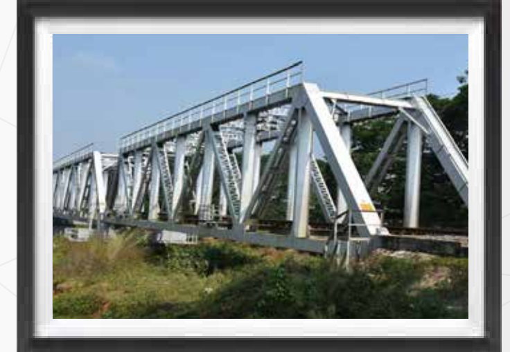
Bridge, East Coast Railways BHUBANESWAR
