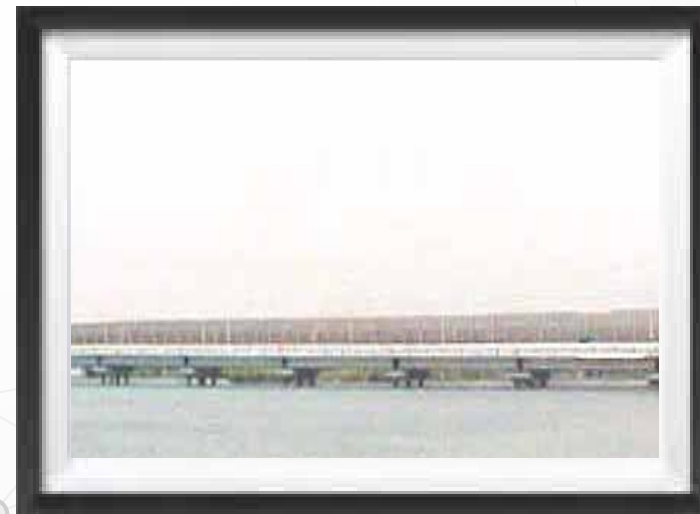
T Girder Bridge VIZAG
