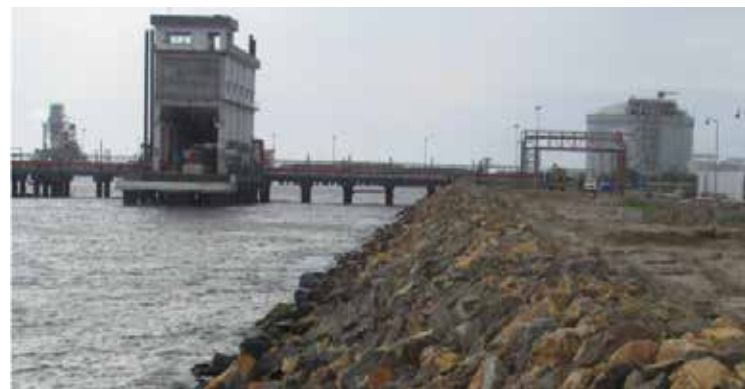
Fire fighting facility and Barge Jetty at Haldia, West Bengal
