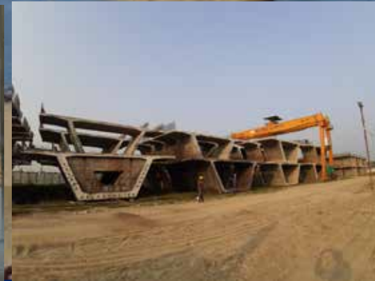
Four Lane Bridge over River Ganga down stream of Farakka Barriage
