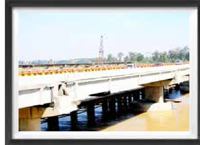
Bridge on River Beas PUNJAB
