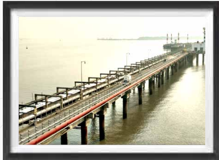
Offshore Berth at Mumbai Port Trust
