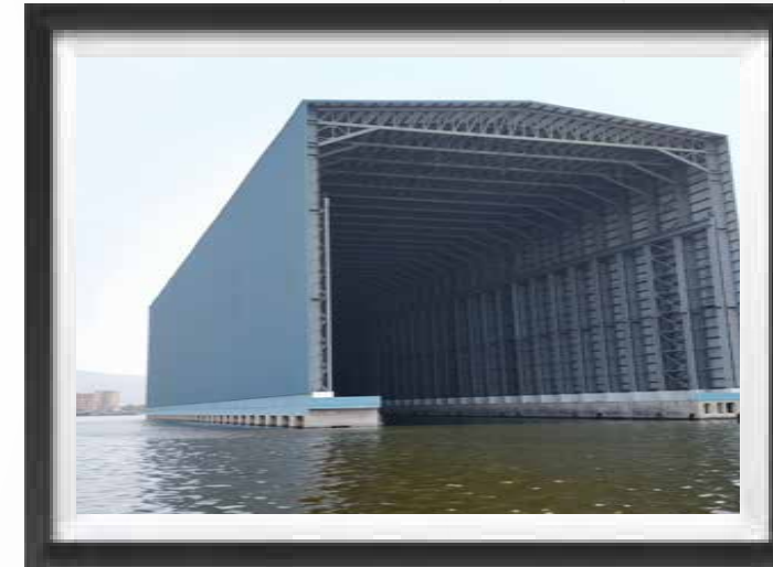
Jetty with loading facility
