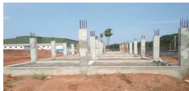
Warehouse for Indian Navy, Vishakhapatnam
