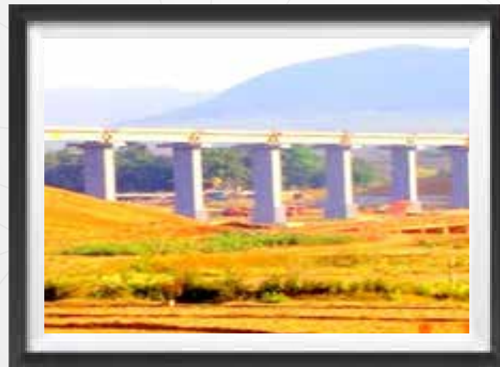
Major Bridge 382, East Coast BHUBANESWAR
