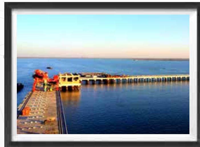
Offshore Berth, Essar Projects
