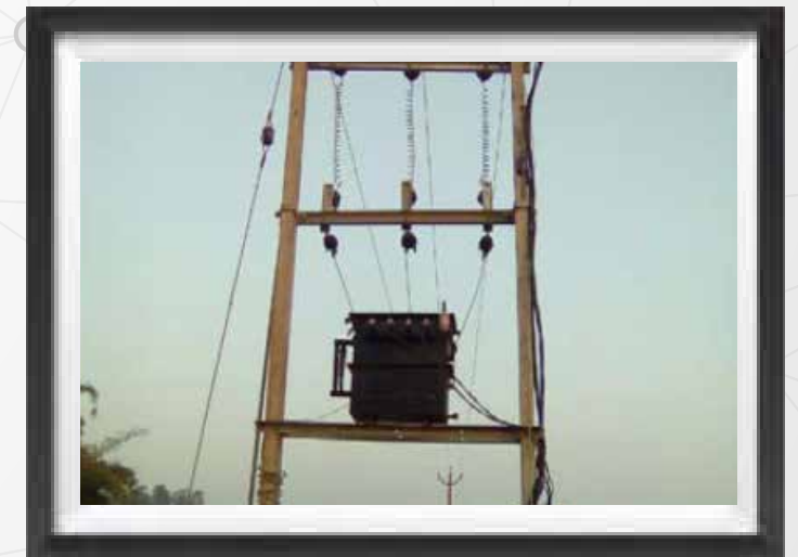
Rural Electrification Work PRATAPGARH
