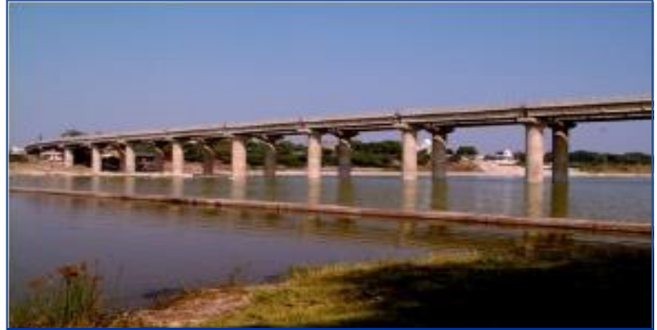
BRIDGE CONSTRUCTION WORK
